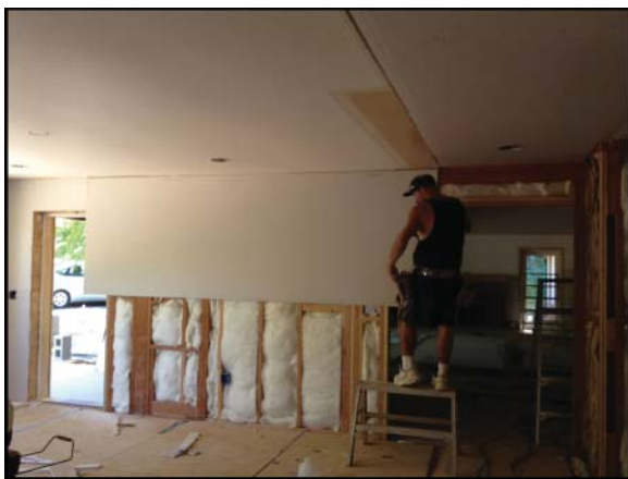
"Sheetrocking" Nevada City Photo by Susan Solinsky
