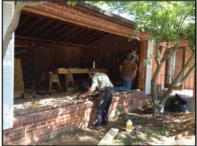
“Front Window Upgrade” Zion Center, Nevada City Photo by Susan Solinsky
